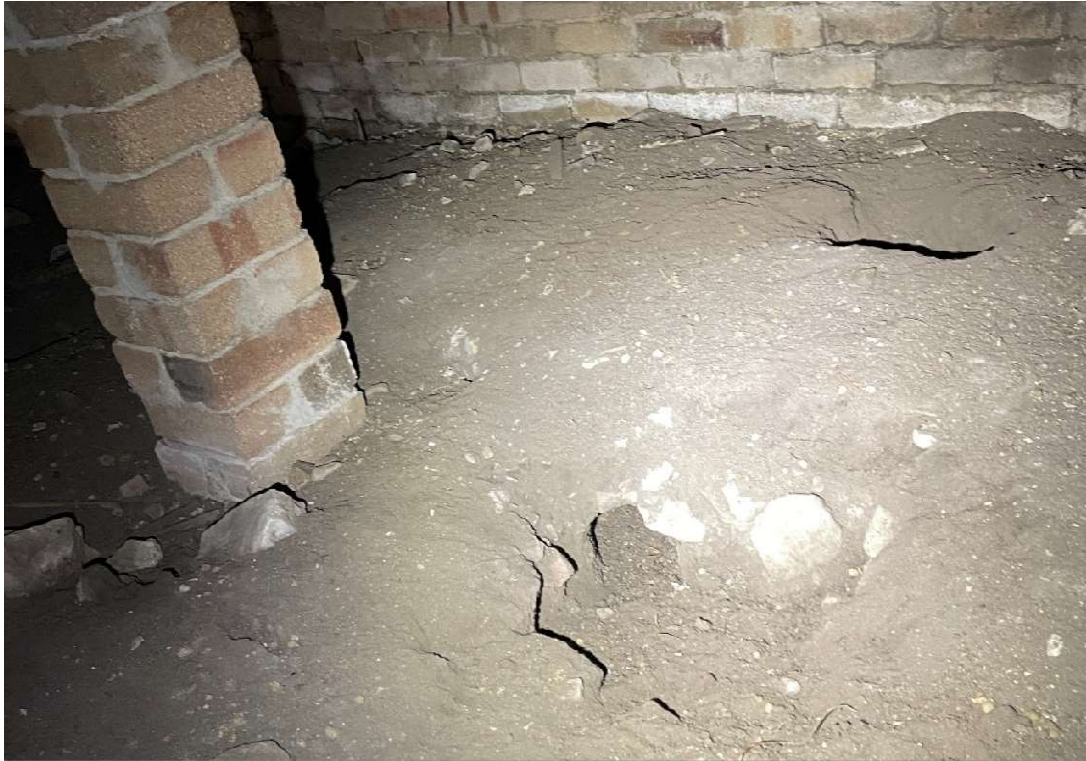
Figure 8 – Sub Floor footing conditions. Animal tunnelling evident in vicinity of brick pier. Structural impact and settlement to footing unclear without further investigation.
