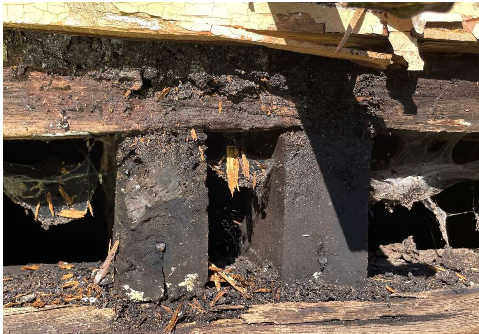
Figure 15 – Close-up of Timber Floor joists at external face of building. Timber is damp likely due to constant water exposure from failing gutter system.
