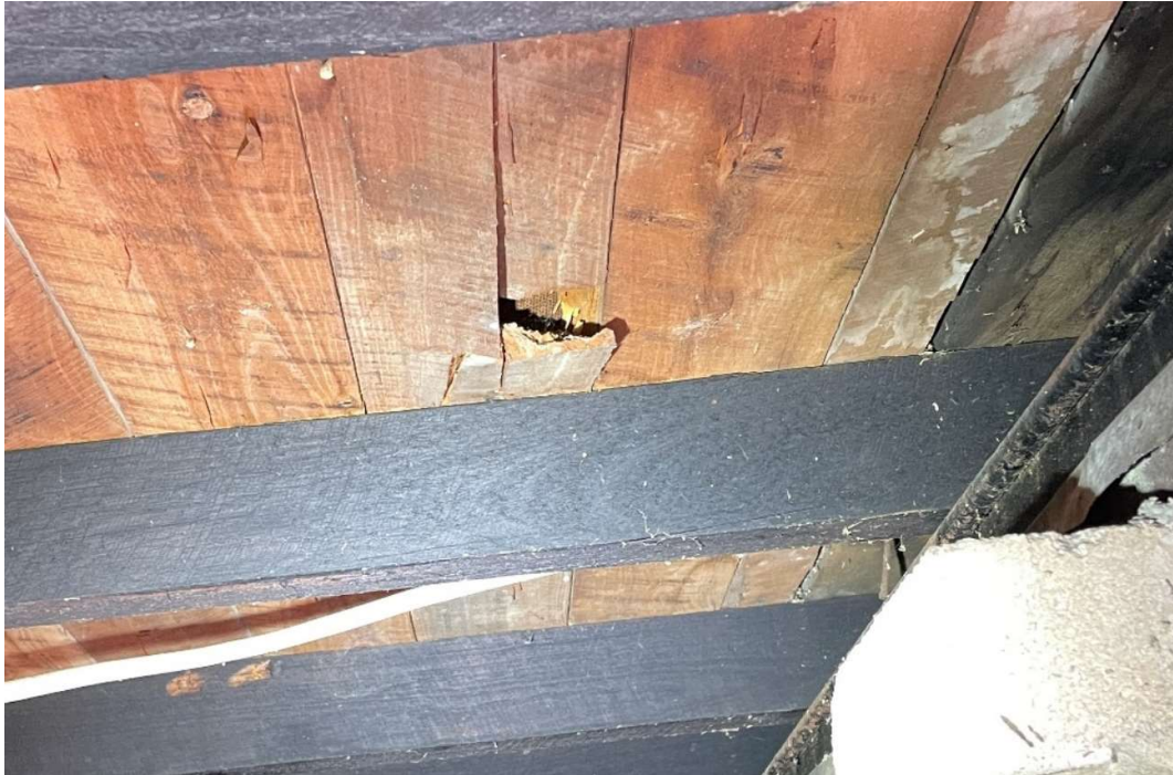
Figure 9 – Localised damage to timber floor plank due to possible overloading.
