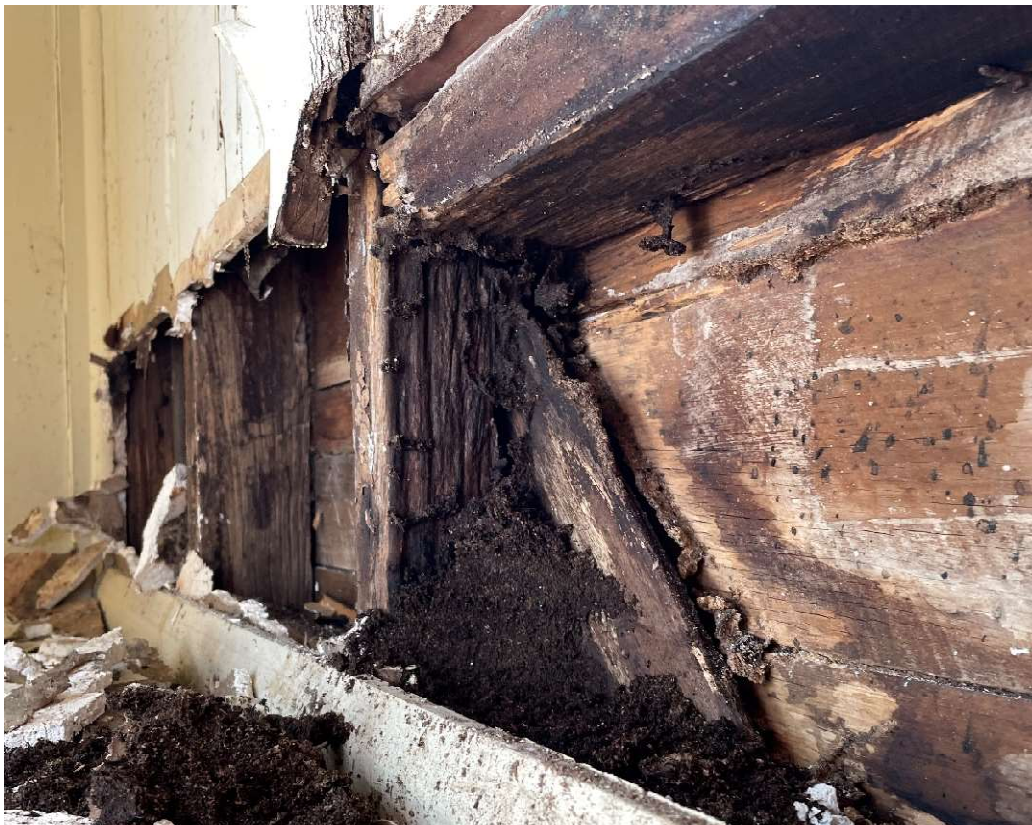
Figure 19 – Timber Stud-Wall at mid-landing of timber stairs joining 2 storeys. Insect faeces at base of studwall indicate likely termite activity within studwall.
