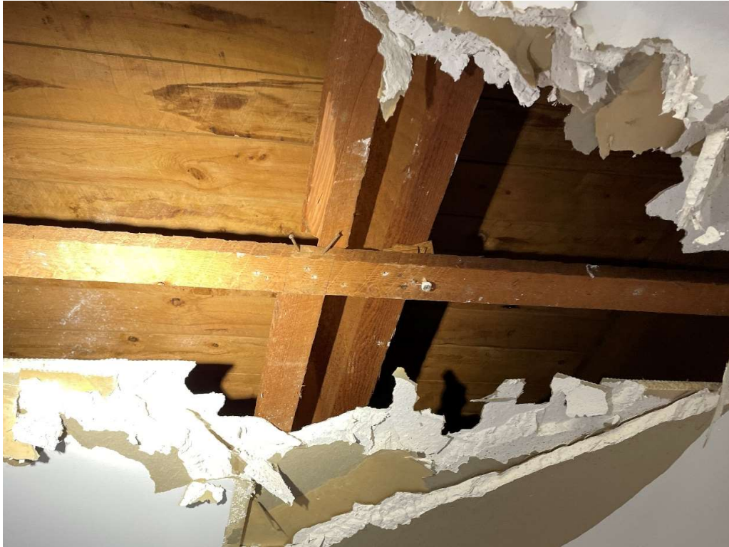
Figure 21 – Typical view of Upper Level Floor framing. No obvious signs of significant weathering or structural defect at this location.
