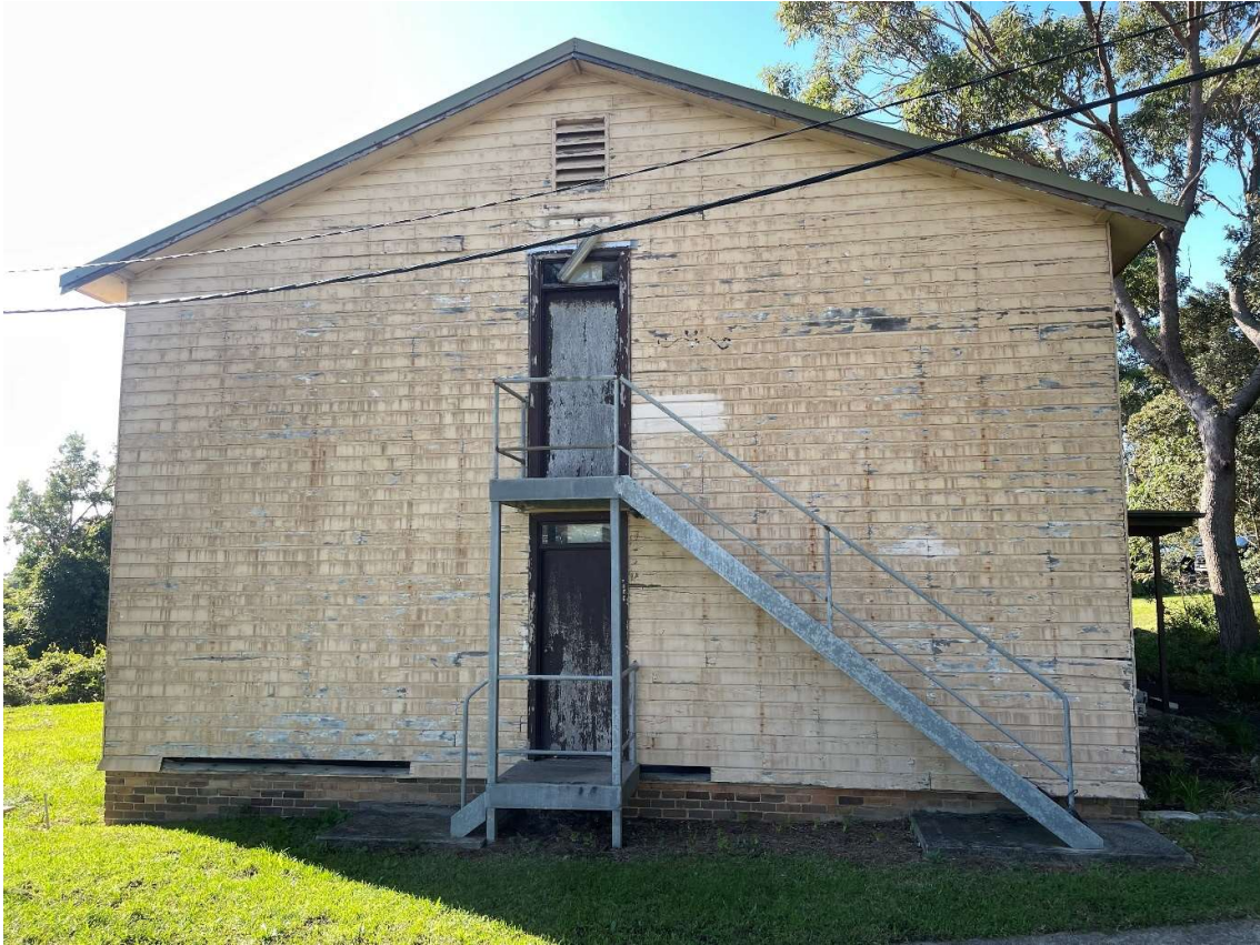
Figure 4 – Typical Side View of Barracks. Gable Style Timber Framed Roof with metal sheeting. Weathering of timber cladding paint system evident.
