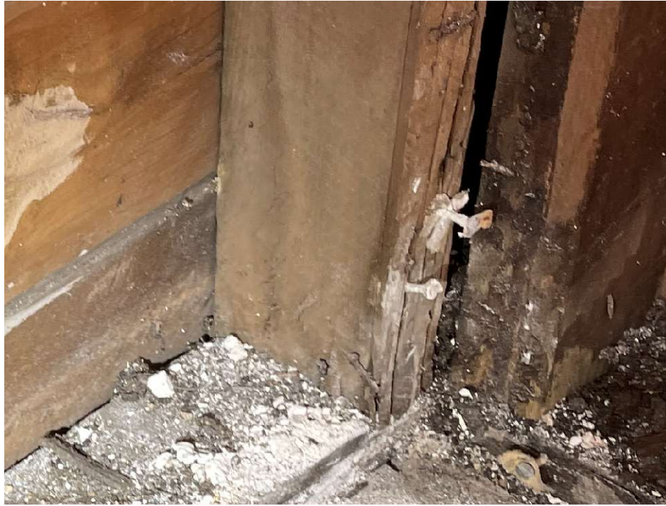
Figure 16 – Internal timber stud-wall. Splitting of timber stud members apparent at ends of studs
