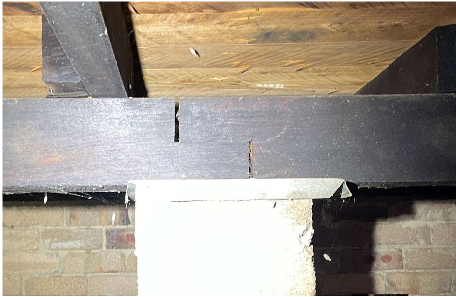
Figure 14 – Timber Flooring beams on brick pier footings supporting floor joists. Vertical cuts in floor beams at support leading to reduced capacity.
