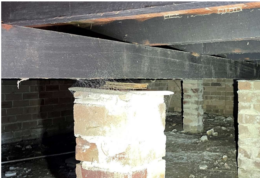
Figure 13 – Existing Sub-floor timber framing. Asbestos packers not engaged with brick pier due to dislodgement of packers or possible footing settlement.
