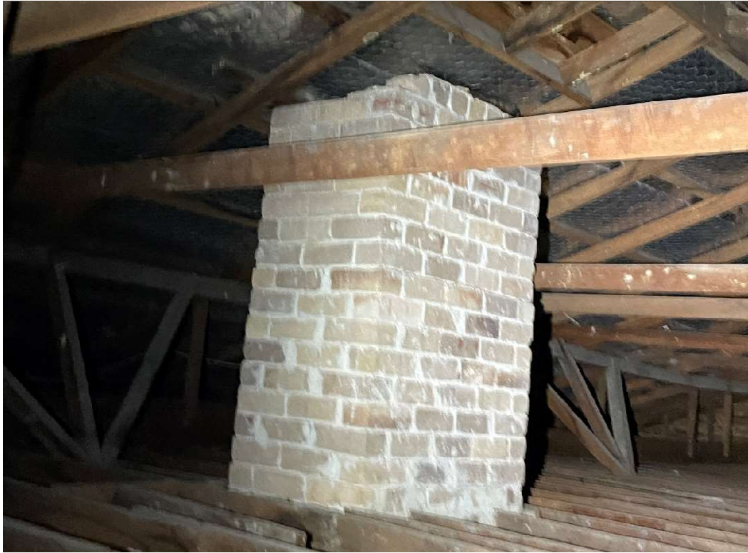
Figure 18 – Non-serviceable Brick chimney terminating within roof structure.
