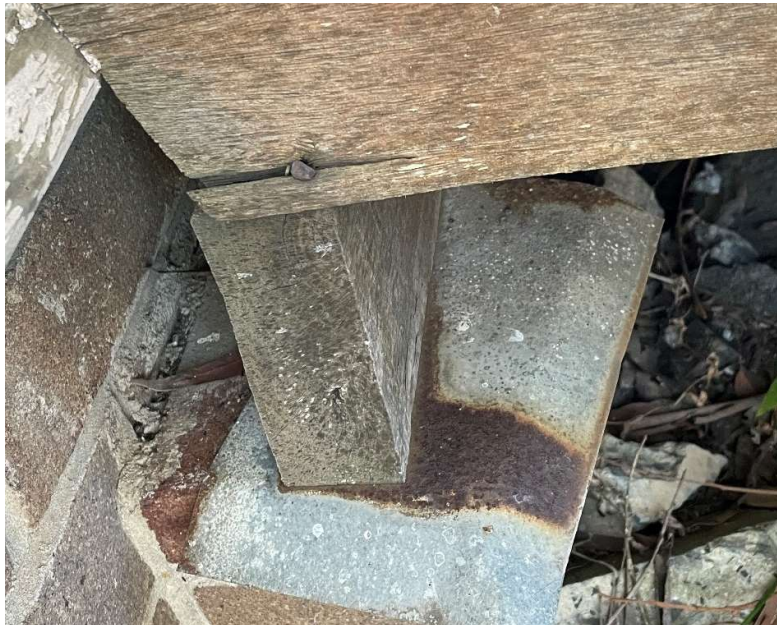
Figure 7 – Close-up of front porch timber floor framing bearing on brick footings. Long-term corrosion of nail evident leading to splitting of timber ends.
