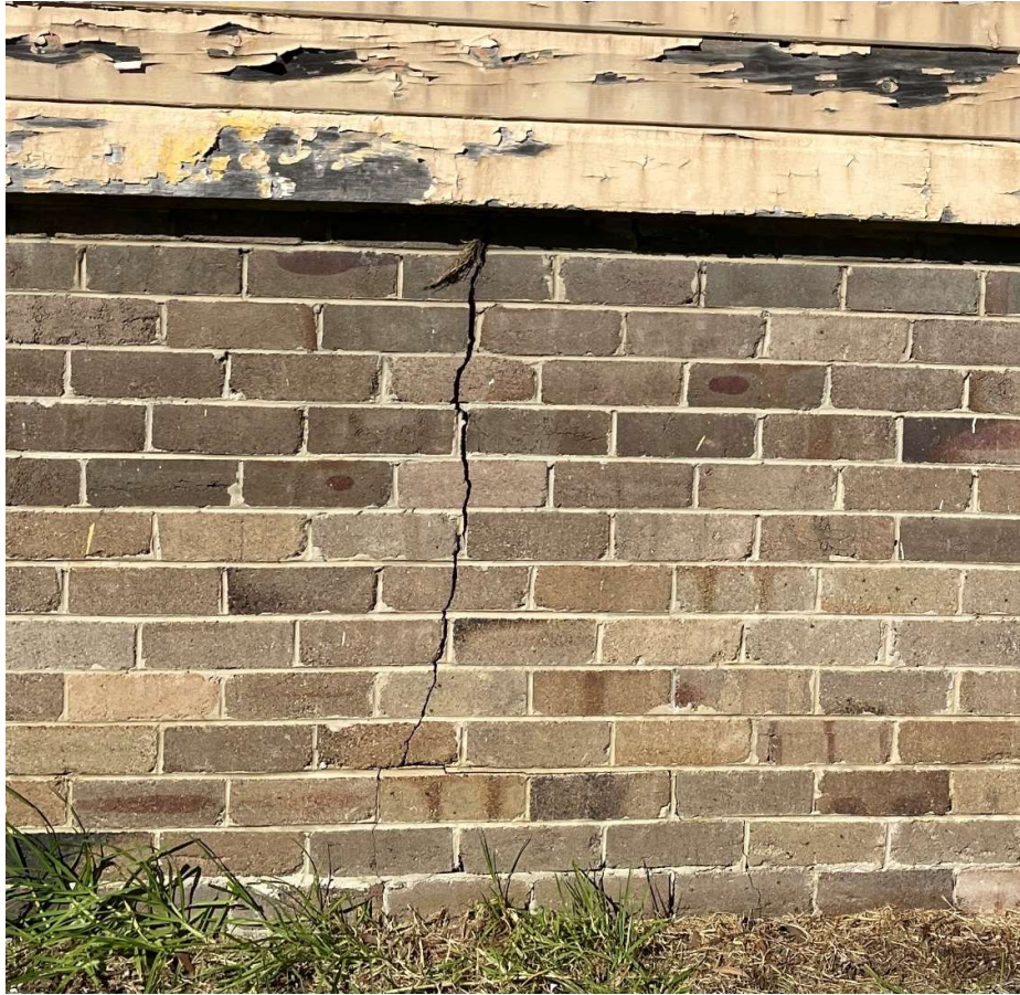
Figure 10 – Vertical Crack in Perimeter Brick Footing Structure due to possible footing settlement.
