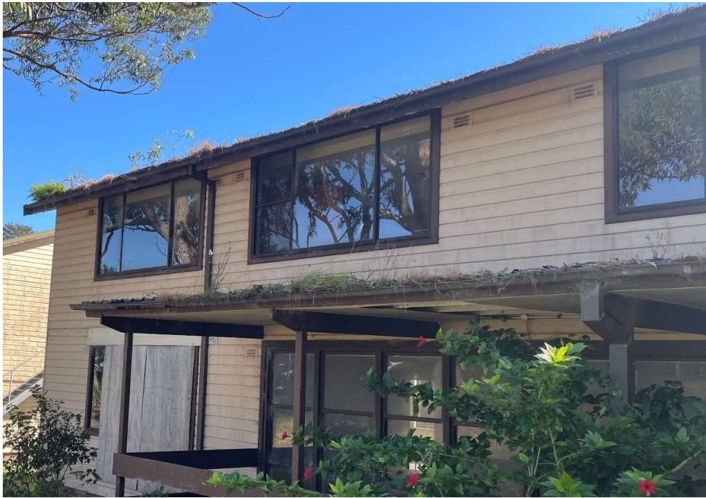
Figure 2 – Typical Front View of Barracks with Front Porch Shelter. Growth within gutters at edge of roof typical
