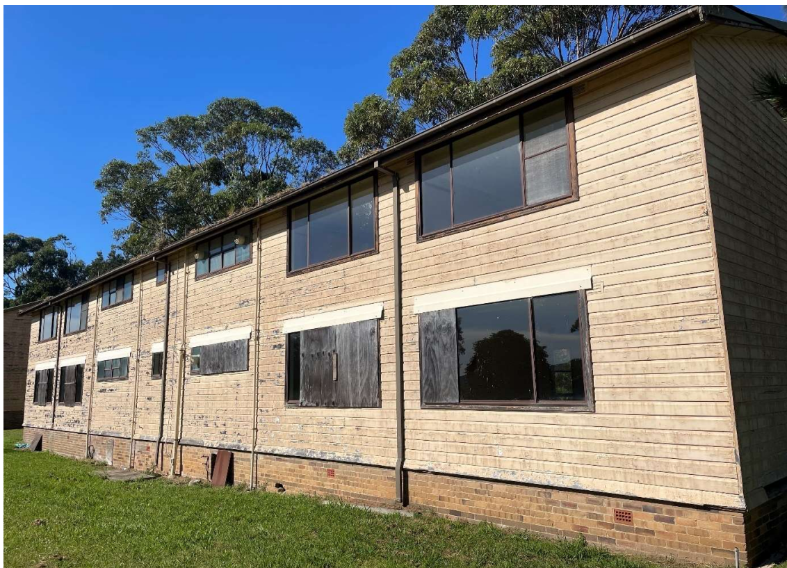
Figure 3 – Typical Rear View of Barracks. Timber weather board-cladding conceals timber studwall on perimeter brick footings for sub-floor framing.
