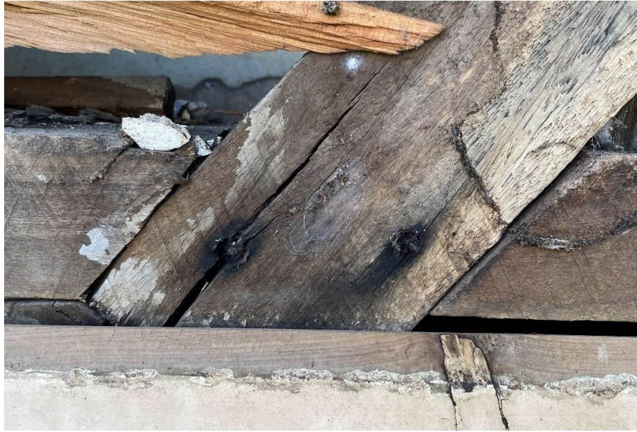
Figure 6 – Close-up of diagonal bracing member junction with perimeter Timber-Framed Wall Bottom Plate. Long-term corrosion of nails evident leading to splitting of timber ends.
