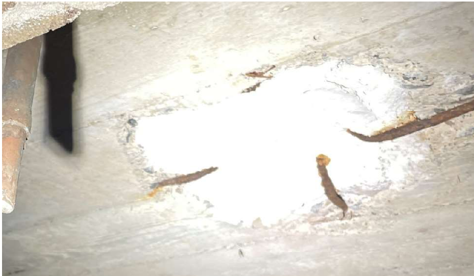
Figure 11 – Cementitious patchwork to underside of existing concrete bathroom slab. Reinforcement bars exposed and indicate surface corrosion.
