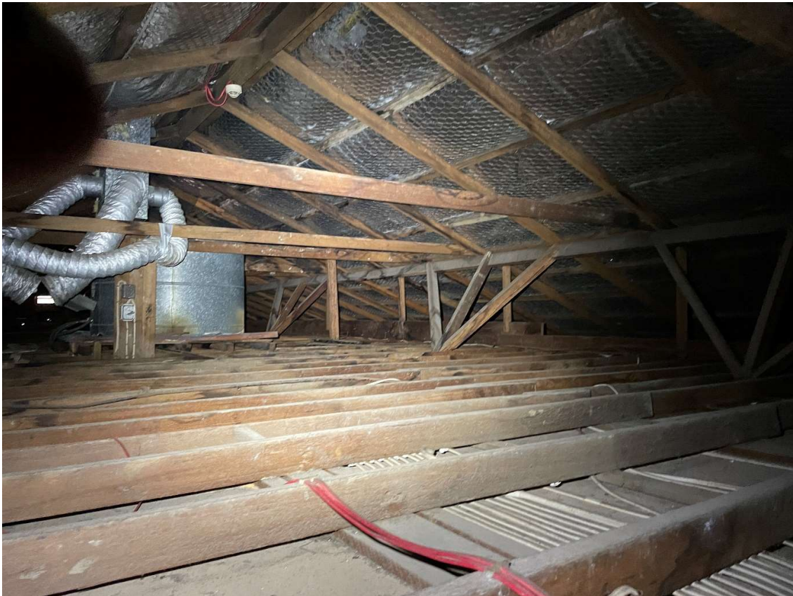
Figure 17 – Typical view of internal gable roof-structure. Sarking, metal mesh, sheeting appear to have been replaced within last 10-15 years. Roof/ceiling structure mostly in good condition.
