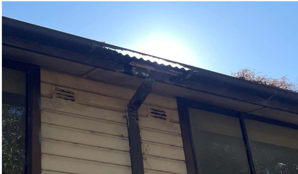
Figure 5 – Gutter Fully corroded through near downpipe due to likely pooling of water and failed drainage.
